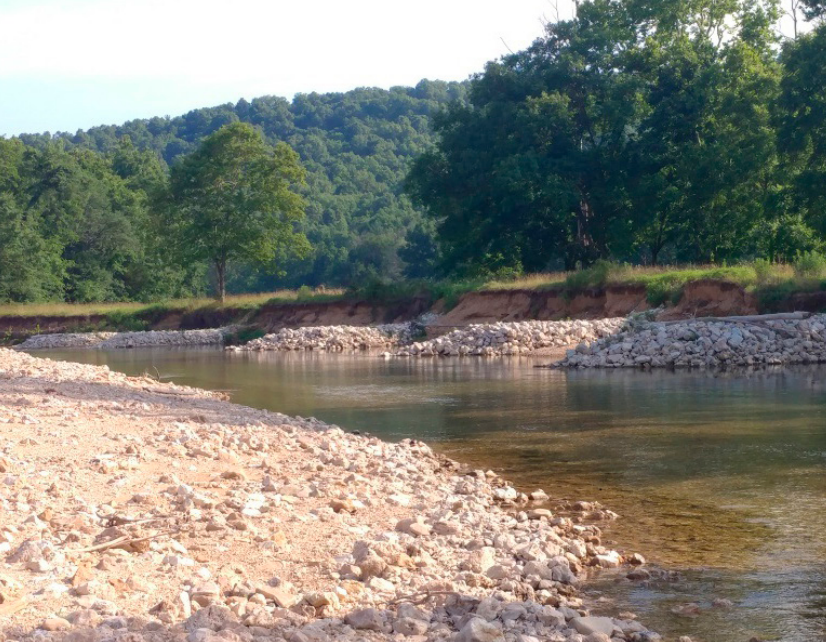
C650 Streambank Stabilization
