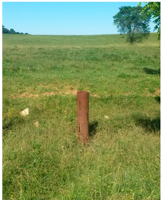
DSP-31 Sinkhole Improvement: Vertical Drain
