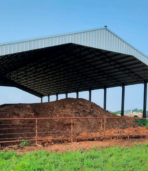
N312 Poultry Waste Management: Stack Shed
