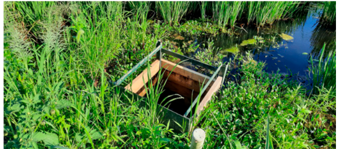
N587 Structure for Water Control-Weirbox
