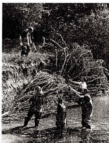
MDC Staff installing the cedar trees on Gabriel Creek.
