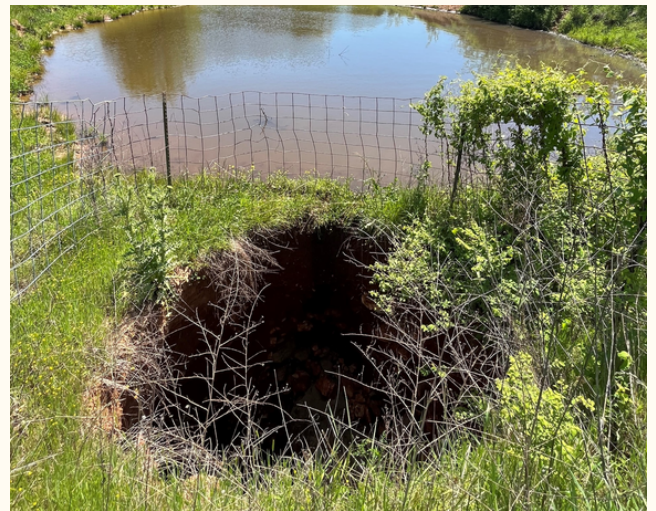
Picture 2: Sinkhole located in Polk County, Missouri.
