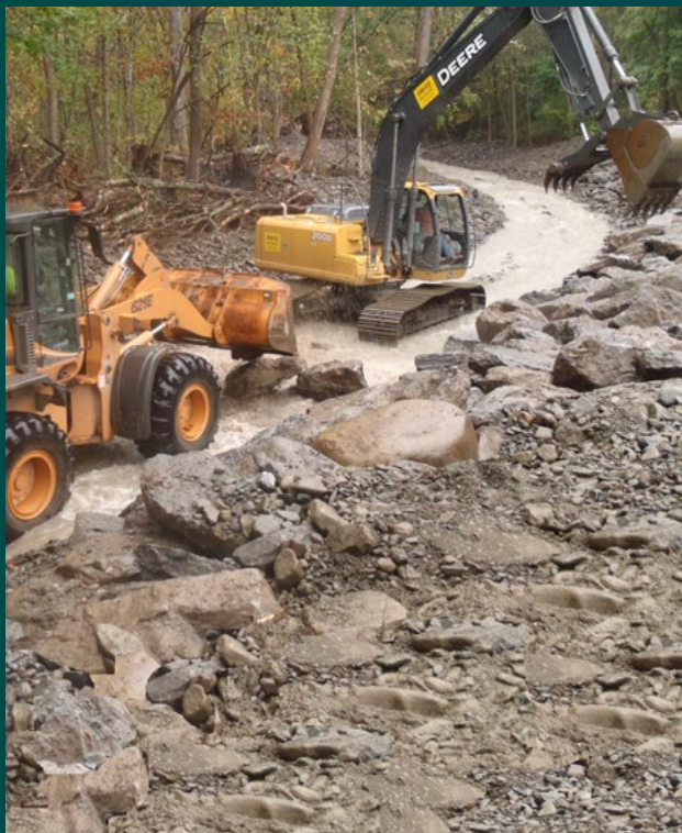
Construction in stream, The Fly Line
